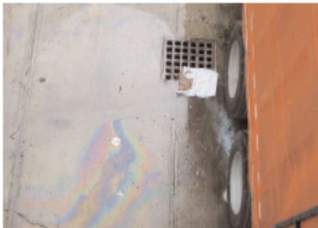
Oil left by parked vehicles will eventually drain to a storm drain network and surface water, where it will degrade fisheries habitats.
