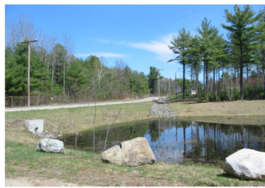
Traditional wet ponds collect heated runoff from paved surfaces and heat it further in the sun before its discharge to a stream. A spillway that discharges through an underdrained gravel trench will cool and slow the release, while offering better pollutant removal efficiencies. The pond can also control peak flows, meeting all four of Maine DEP's objectives.
