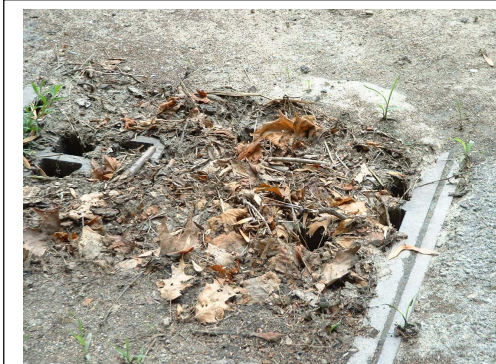
Leaves that enter the storm drain networks are carried into receiving waters, where they use oxygen to decompose. Reduced dissolved oxygen in the water is toxic to aquatic life.
