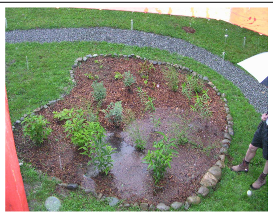
Some communities have reduced the total stormwater load by disconnecting the impervious areas and by building rain gardens. These projects are reducing flooding problems and become an attractive part of the landscape.
